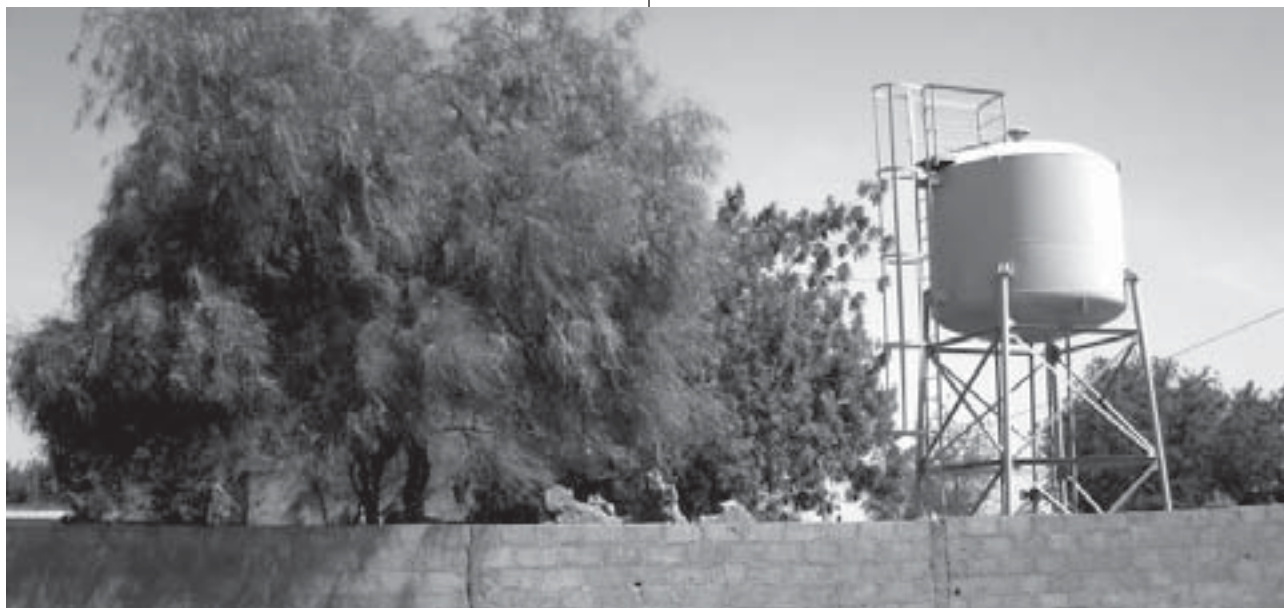
Drinking water conveyance in Fakala.
